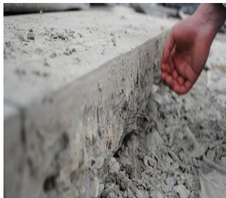
Figure 3. PVA fiber concrete roadbed 图 3. PVA 纤维混凝土路基
