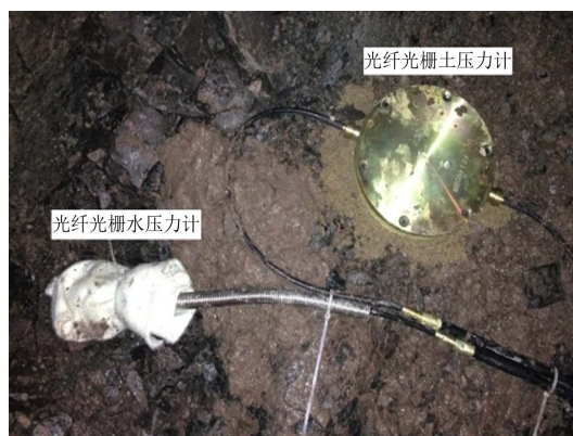
Figure 2. Installing the track bed sensor
