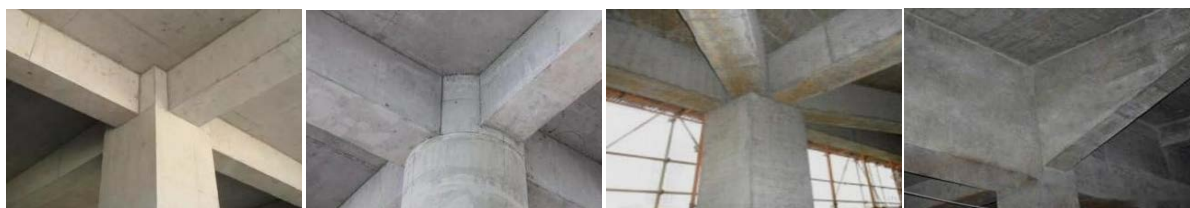
Figure 1. Common beam-column joints in reinforced concrete structures
