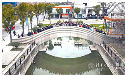
The world's longest 3 D-printed pedestrian bridge
