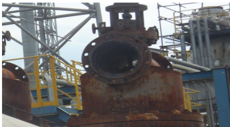
Figure 1. Below is the replacement of the high-temperature mixing valve removed
