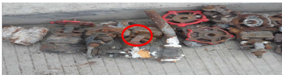
Figure 6. Removing the corroded valve from the exhaust gas treatment
