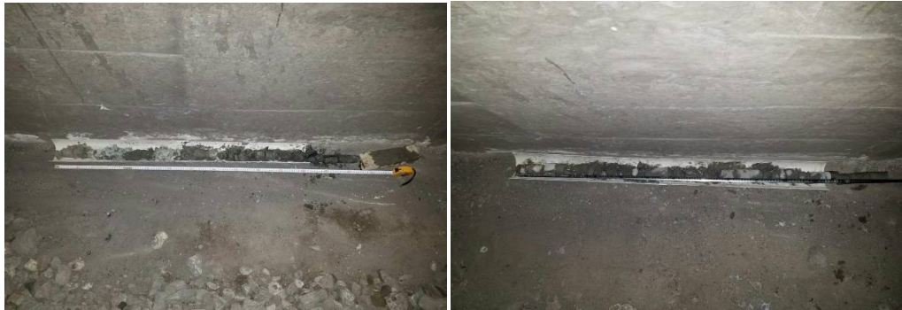
Figure 9. Coring at the bottom of the tunnel 图 9. 隧道底部取芯
