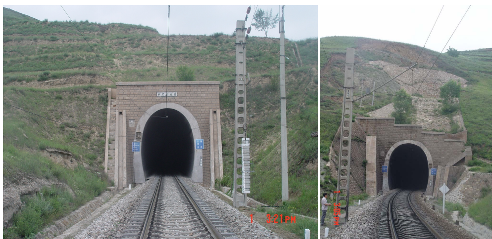
Figure 1. Geomorphic features of Wulishan Tunnel
