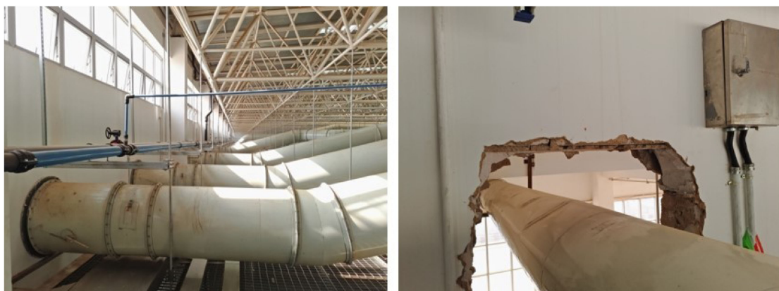
Figure 3. Pipes through the wall
