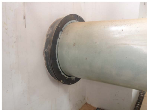
Figure 8. Through-wall pipe clamp installation 图 8. 穿墙管道夹持装置安装
