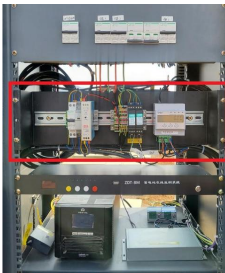
Figure 5. Before the distribution box line rectification
