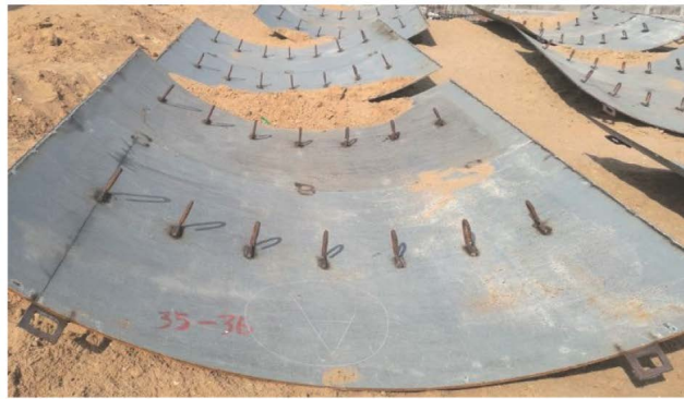
Figure 2. The hook diagram of arc-shaped steel plate hook 图 2. 弧形钢板弯钩图
