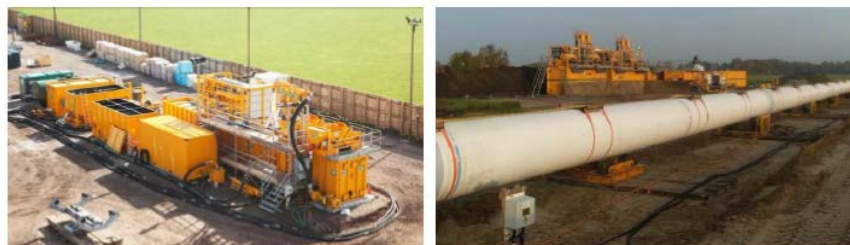
Figure 15. Installation of the mud recycling system 图 15. 泥浆系统安装
