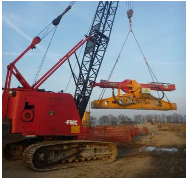
Figure 7. Installation of the hydraulic cylinder 图 7. 单侧底座及推进油缸
