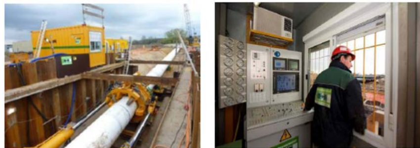
Figure 14. Installation of the control cabin 图 14. 控制室安装
