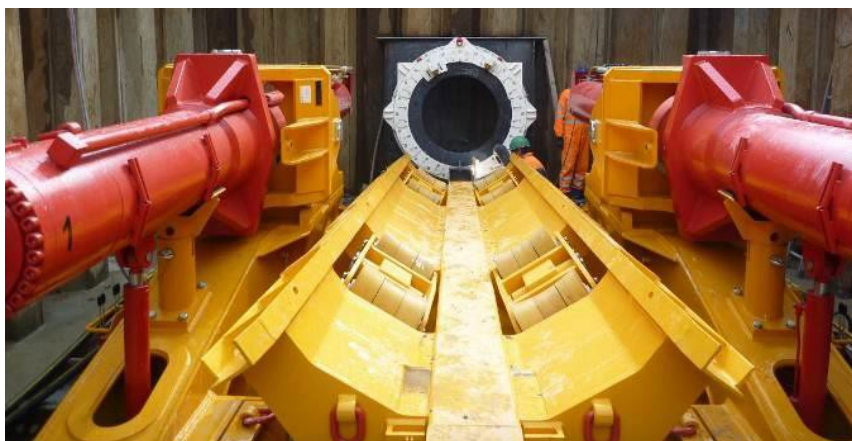
Figure 9. Installation of the launch cradle 图 9. 发送导轨安装
