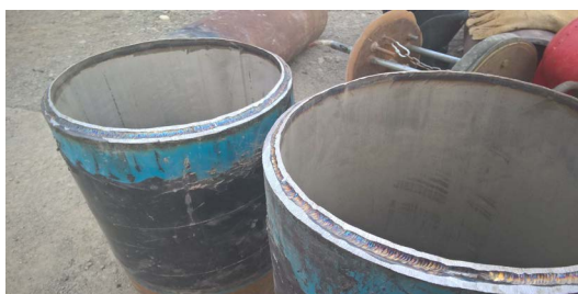
Figure 9. Tube end seal welding 图 9. 管端封焊
