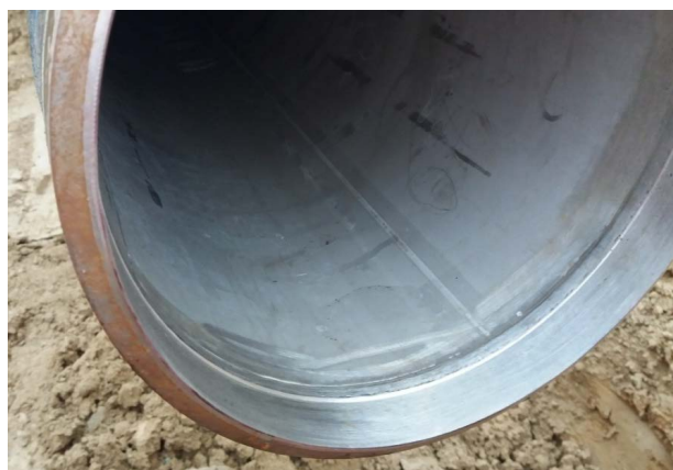
Figure 5. Pipe section sealing 图 5. 管段封焊
