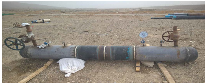
Figure 10. Head pressure test 图 10. 封头试压
