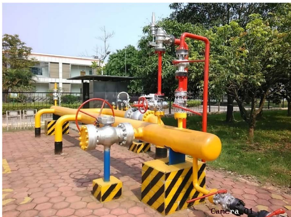
Figure 10. The installation position of orifice plate device in Nanlang station is shown in the frame 图 10. 南朗站孔板装置安装位置如框中
