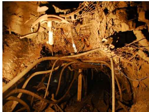
Figure 2. Case of roadway destruction
