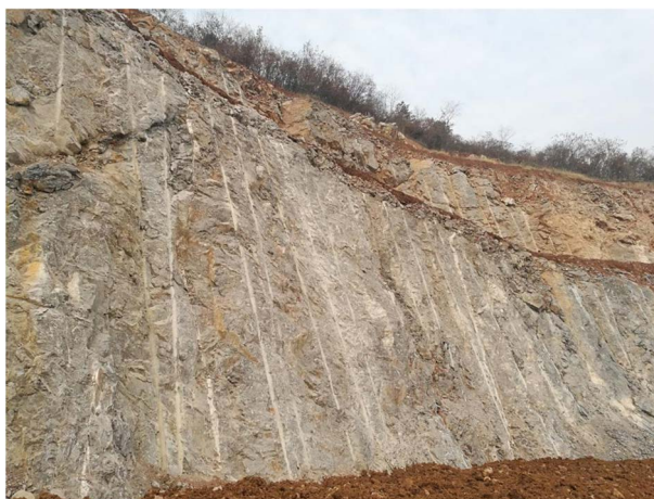
Figure 4. Smooth surface of pre-split controlled blasting slope 图 4. 预裂控制爆破边坡光面情况
