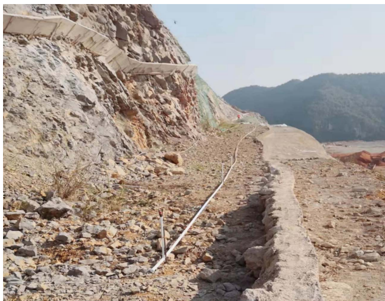
Figure 3. Slope V-groove and step planting groove 图 3. 边坡 V 形槽及台阶种植槽
