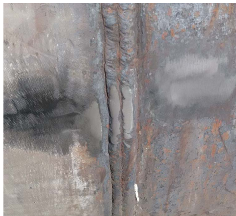
Figure 5. Welds hardness polishing 图 5. 焊缝硬度打磨
