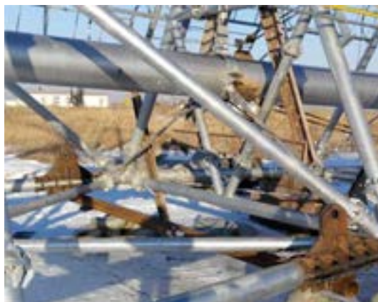
Figure 13. Strengthening of the lifting lug 图 13. 溜尾吊耳加固
