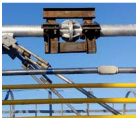
Figure 15. Strengthening of the column of the flange 图 15. 立柱法兰加固
