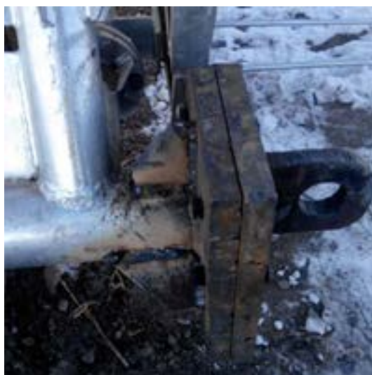
Figure 14. Strengthening of the primary lifting lug 图 14. 主吊耳加固
