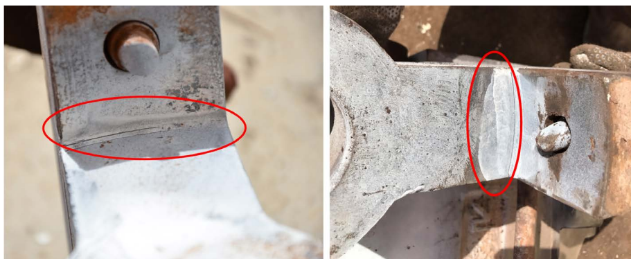
Figure 2. Details of crack at shoulder root of elevator latch 图 2. 吊卡卡页台肩根部裂纹细节图
