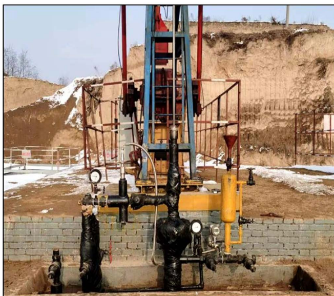
Figure 7. Field application of Guping 30-21 well 图 7. 固平 30-21 井装置现场应用
