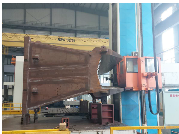
Figure 5. The actual situation of the processing of the saddle cable groove of the loose cable 图 5. 散索鞍索槽加工实物情况
