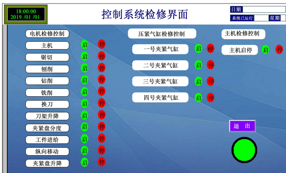
Figure 5. Multi-station beam and column furniture components forming machine control system maintenance interface
