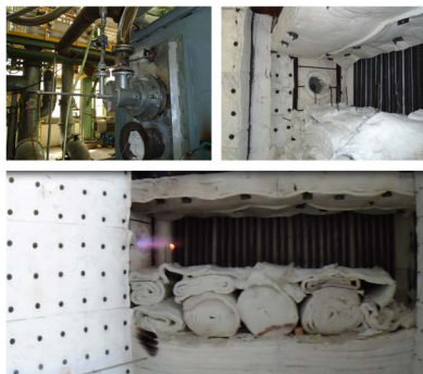
Figure 4. Pictures of IHVB type burner after installation
