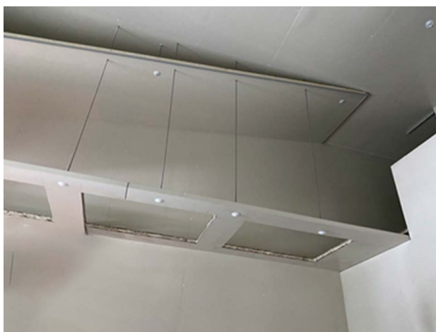
Figure 9. Air supply duct structure 图 9. 送风风道结构
