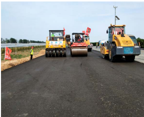
Figure 7. Compaction of cold mix and cold paving asphalt mixture 图 7. 冷拌冷铺沥青混合料压实
