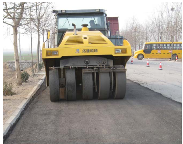
Figure 6. Cold mix cold paving asphalt mixture paving 图 6. 冷拌冷铺沥青混合料摊铺
