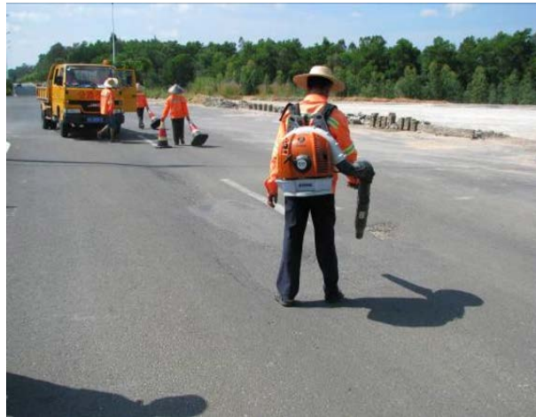
Figure 5. Cleaning of lower bearing layer 图 5. 下承层清扫
