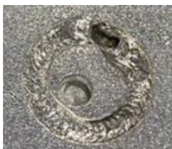
Figure 10. Weld surface hole defect
