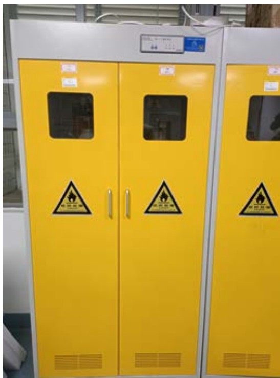
Figure 2. The explosion-proof cabinets are used to store steel bottles in laboratory
