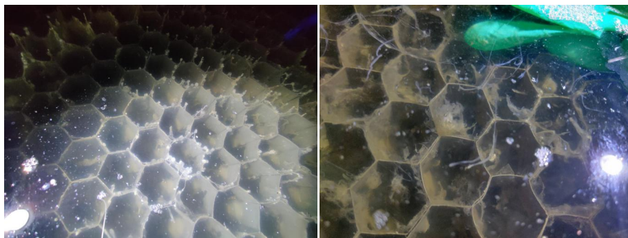
Figure 15. Comparison of bacterial membrane state in denitrification tank before and after drug adding
