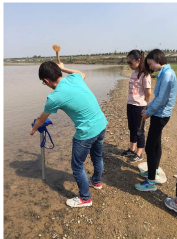
Figure 2. Recorder installation 图 2. 记录仪安装
