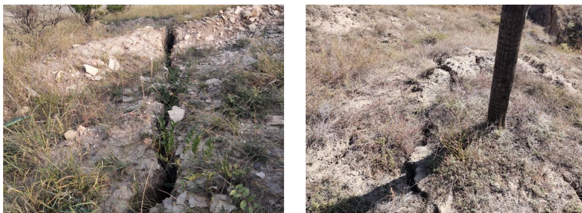
Figure 2. Field investigation of ground fissures 图 2. 实地调查地裂缝
