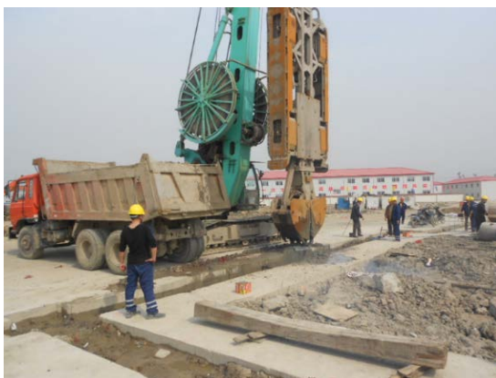
Figure 4. Trench section excavation construction site 图 4. 槽段开挖施工现场图
