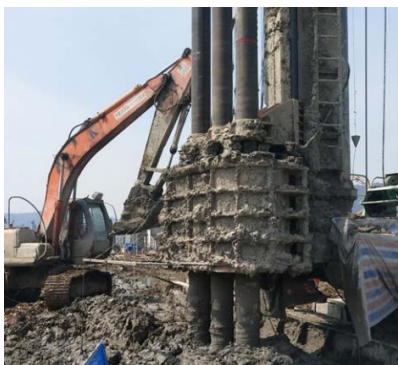
Figure 3. Tri-axial mixing pile construction site 图 3. 三轴搅拌桩施工现场图
