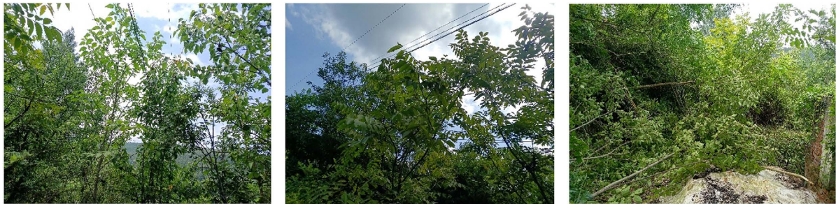
Figure 3. Wild trees and miscellaneous trees endanger power lines 图3. 野树杂木危及电线
