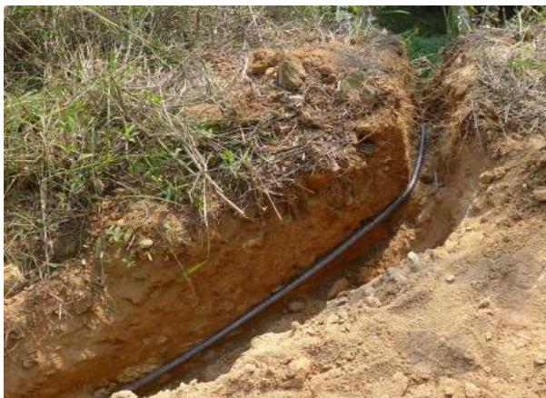
Figure 1. Flexible graphite composite grounding material 图 1. 柔性石墨复合接地材料
