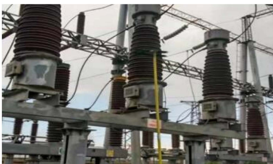
Figure 13. Cleaning of ceramic contamination processor in practical environment 图 13. 实际环境下瓷瓶污秽处理器清扫工作
