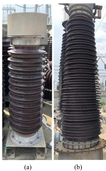
Figure 5. Insulators of two different sizes 图 5. 两种不同尺寸的瓷瓶
