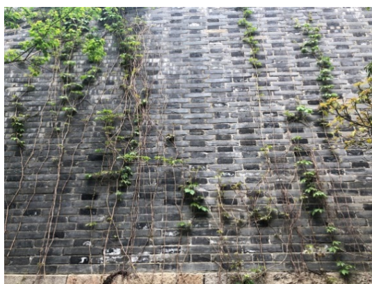
Figure 4. Surface of the wall
