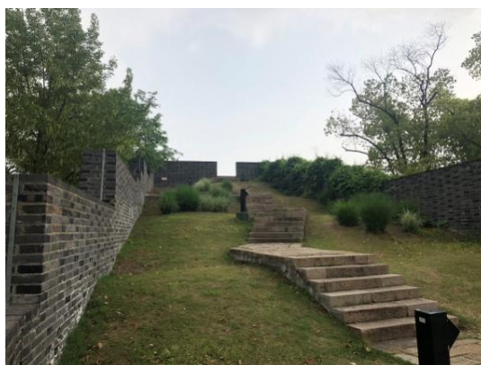
Figure 3. Soil on the top of the wall
