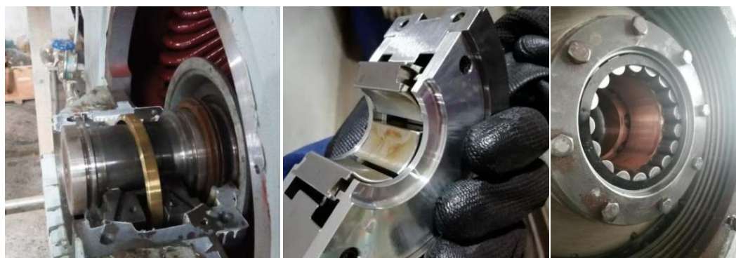
Figure 3. Explanation of the structure and function of the parts in the disassembly drawing of the bearing seat
