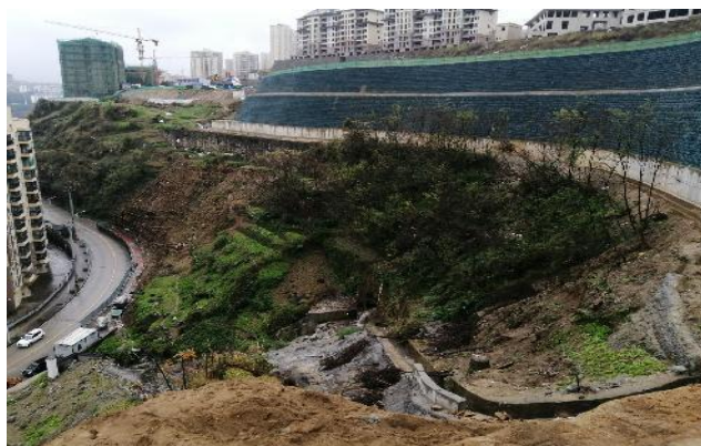
Figure 1. Photo of the parallel segment
