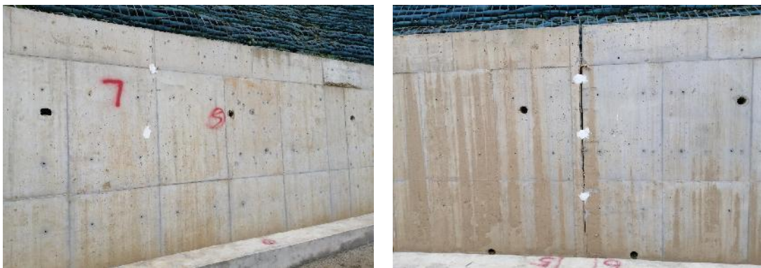
Figure 2. Crack in the left side of the slope
