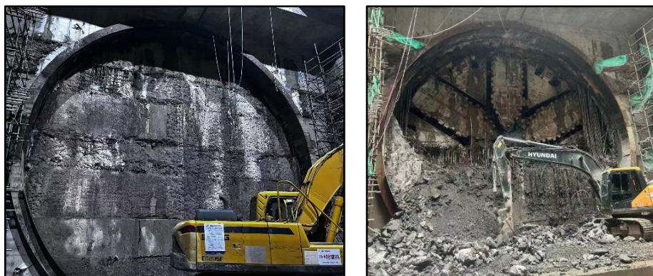
Figure 1. Opening chiseling 图 1. 洞门破除
